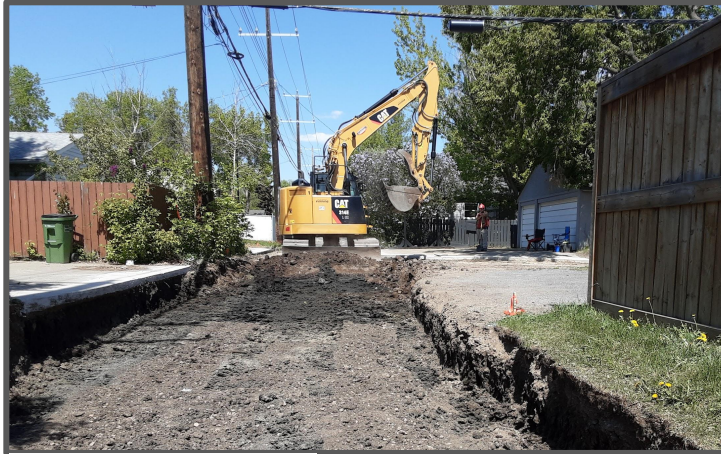
Active Alley Reconstruction
